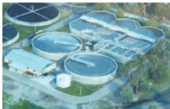
Figure 8.7 An aerial view of a sewage plant
